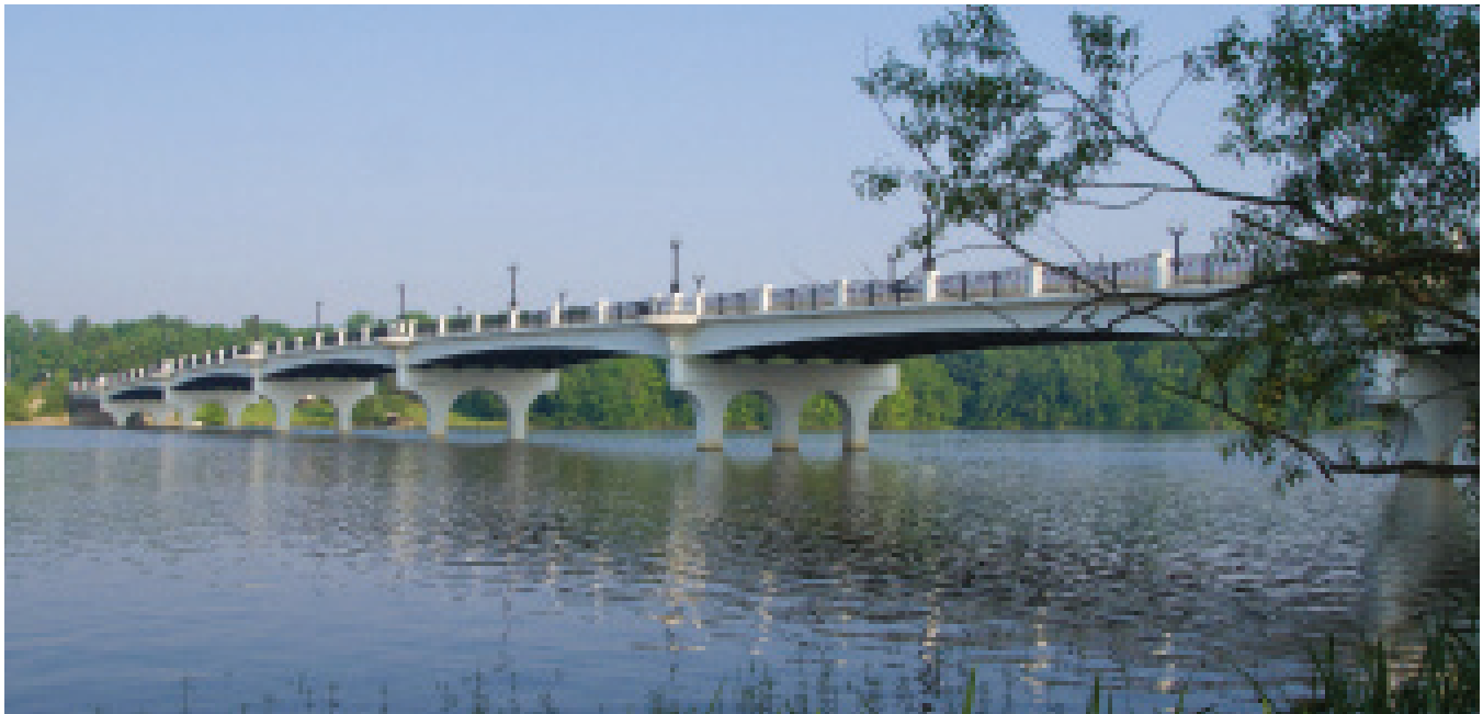
Delaware County Home Road Bridge
